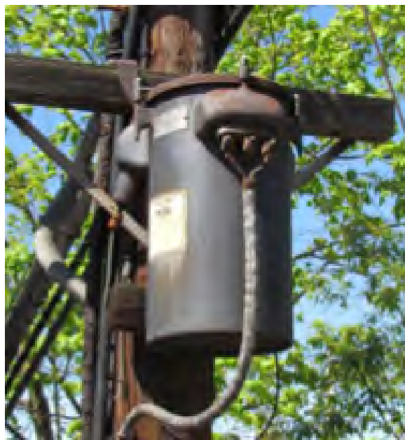
Electrical transformers manufactured prior to 1977 may still contain PCBs. (Photo: Wikipedia)
